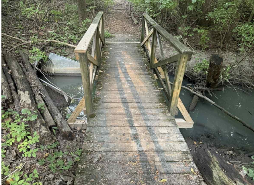
Figure 1. A photo of the current bridge.
