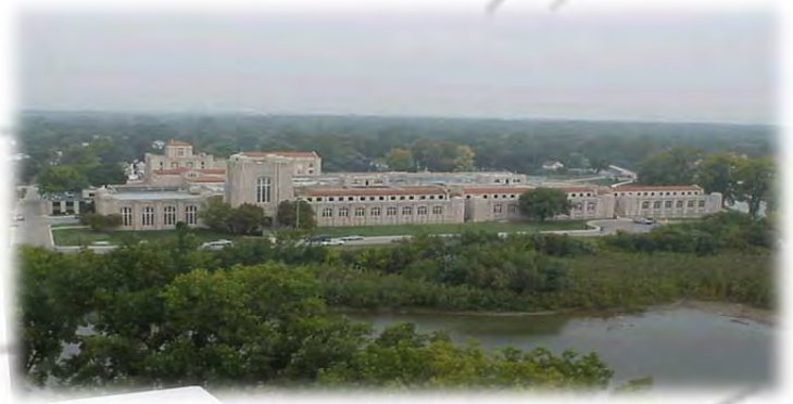
Figure 8: Fort Wayne Three Rivers Filtration Plant
