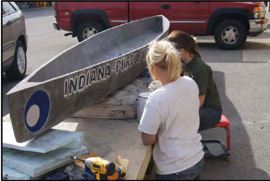
Figure 15: Blue graphic and concrete paint lettering being applied.
