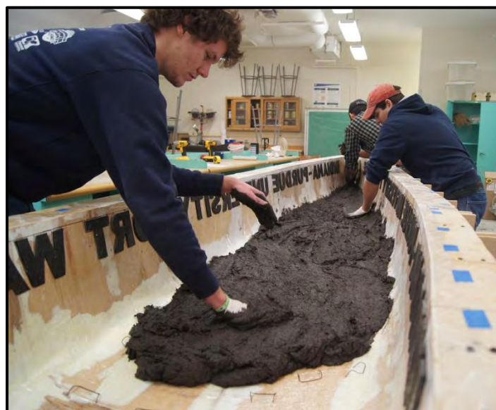
Figure 10: First layer of concrete being placed.
