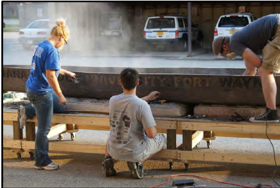
Figure 14: Sanding and removing the inlays.
