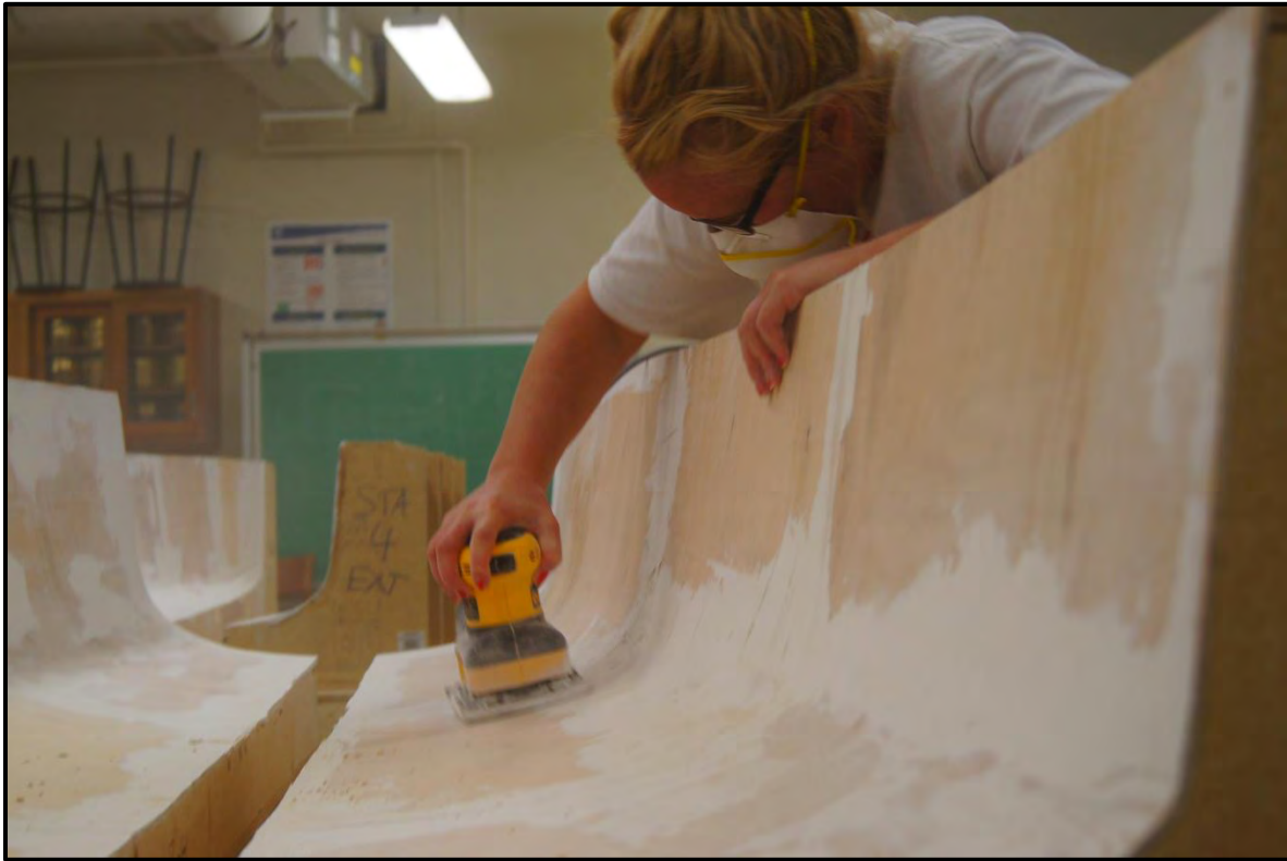
Figure 4: Sanding the wood with the joint compound applied.
