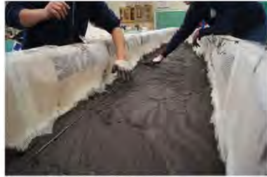
Figure 6: Placement of Reinforcement.
