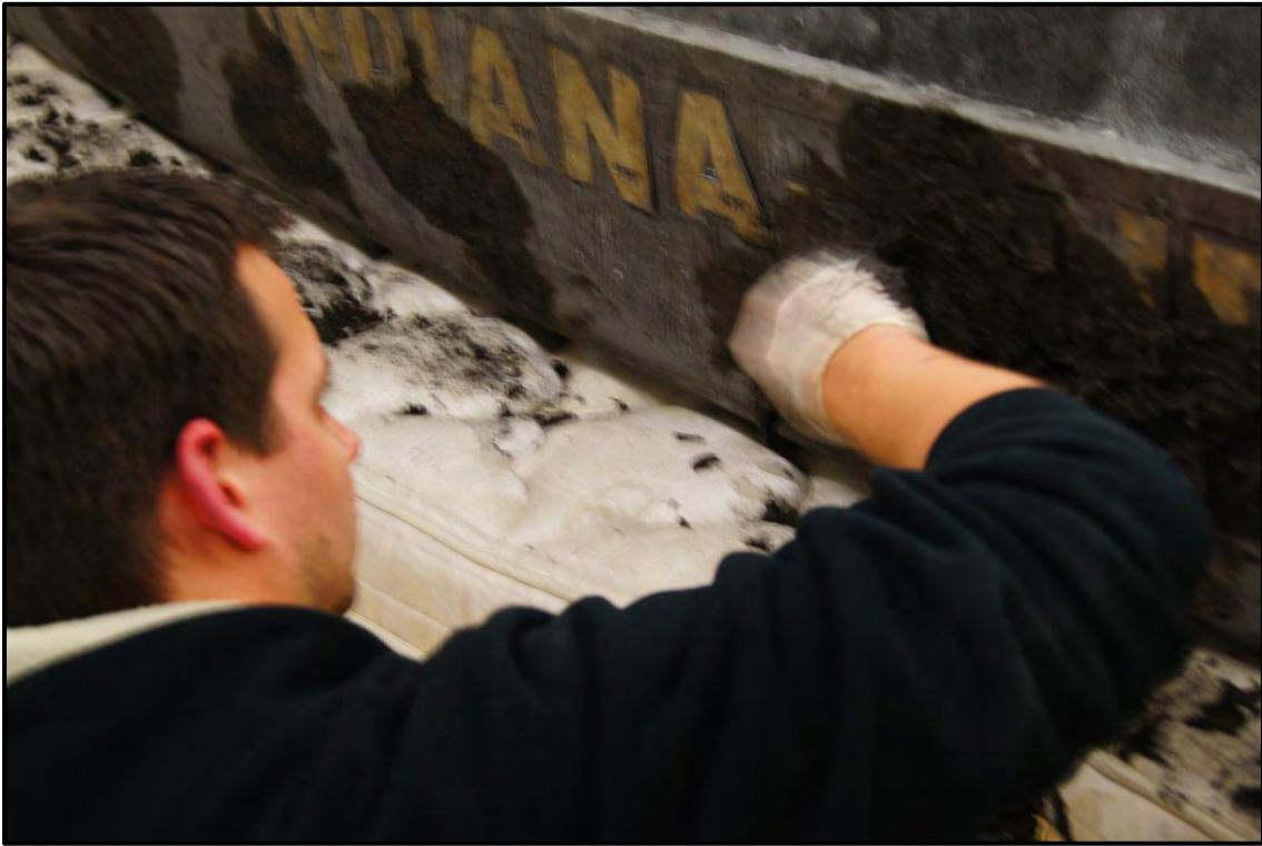
Figure 18: The patch mix being applied where needed.
