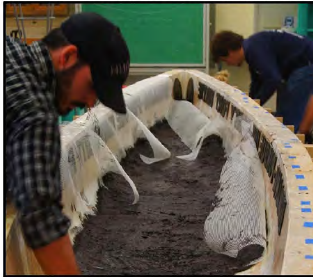
Figure 8: Placing the first layer of fiberglass grid reinforcement and another thin layer of concrete.
